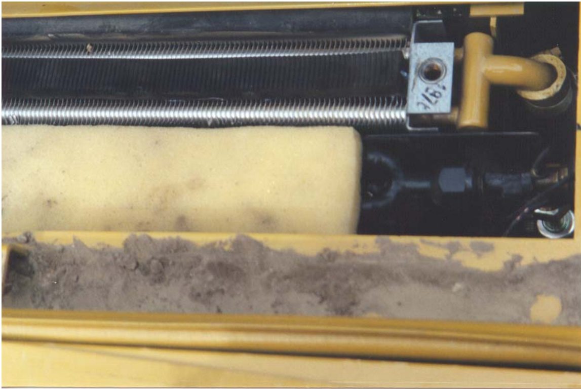
Top of evaporator assembly in heater box.
