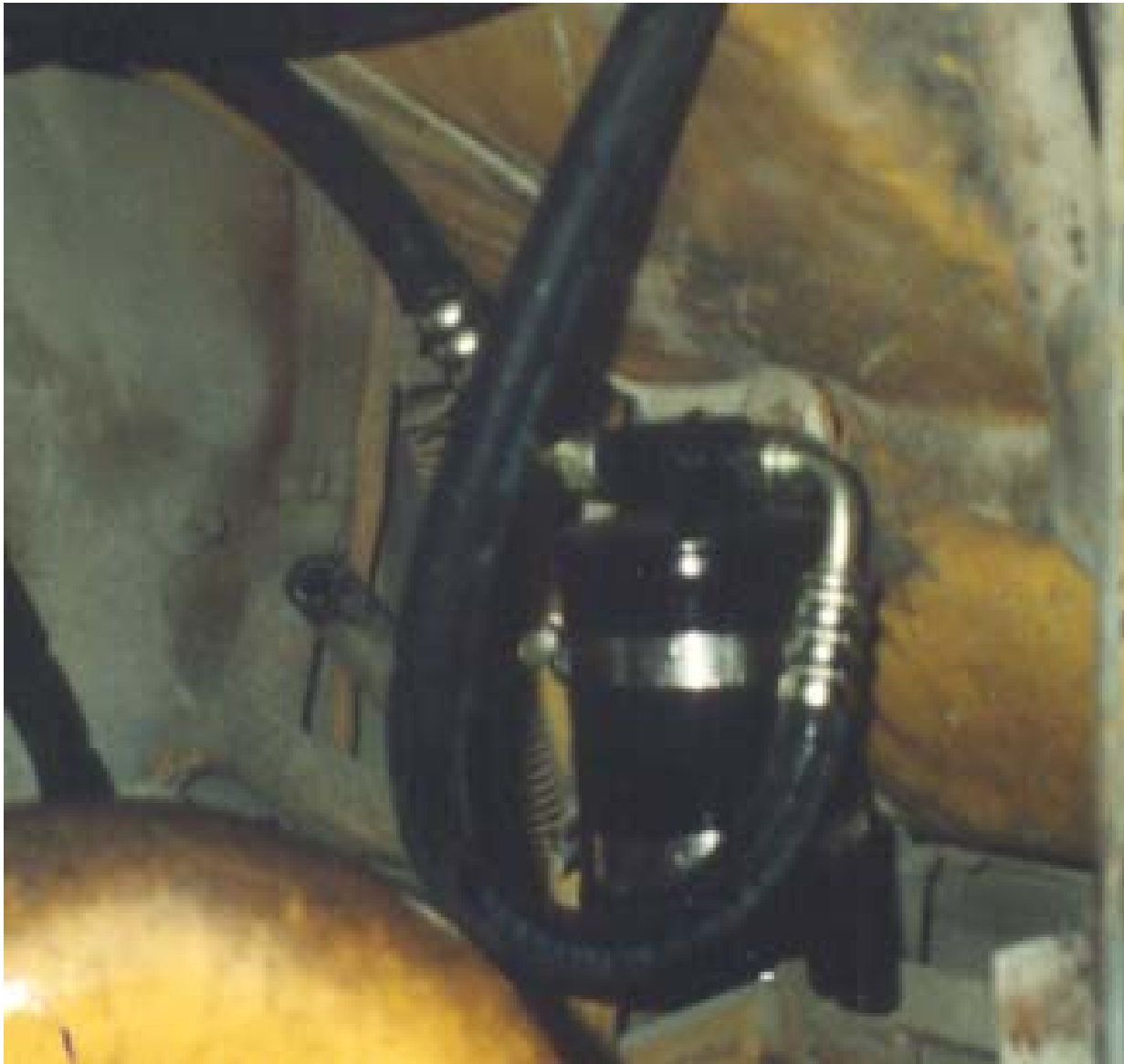
Drier in location with hoses run.
